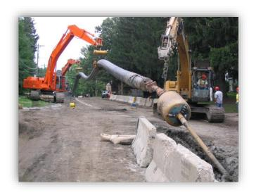
DriscoPlex® HDPE piping is an excellent choice for rehabilitating deteriorated pipelines. Trenchless rehabilitating options include sliplining a smaller HDPE pipe into an existing pipe and pipe bursting, which involves expanding or breaking an existing pipe into the surrounding soil while simultaneously pulling in the new HDPE pipe. See Chapters 11 and 16 of the PPI Handbook of PE pipe for additional information.
